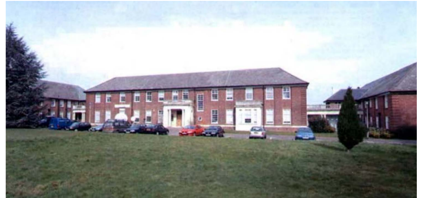
Listed Building- Officers Mess.
