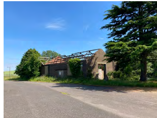
View of derelict former workshops
