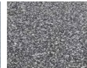
Permeable tarmac - Driveway
