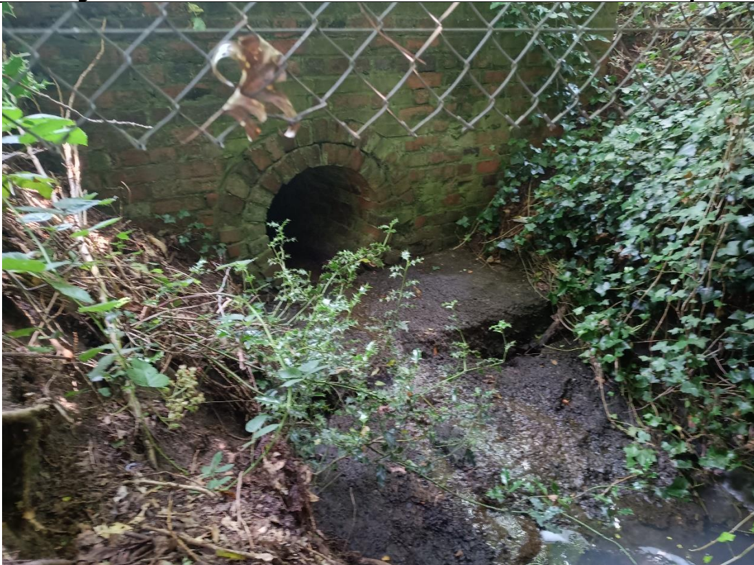
Figure A.5 – Culvert under railway line draining to watercourse within adjacent cemetery
