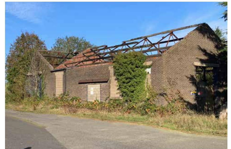
Figure 5.7 Derelict Workshop Building
