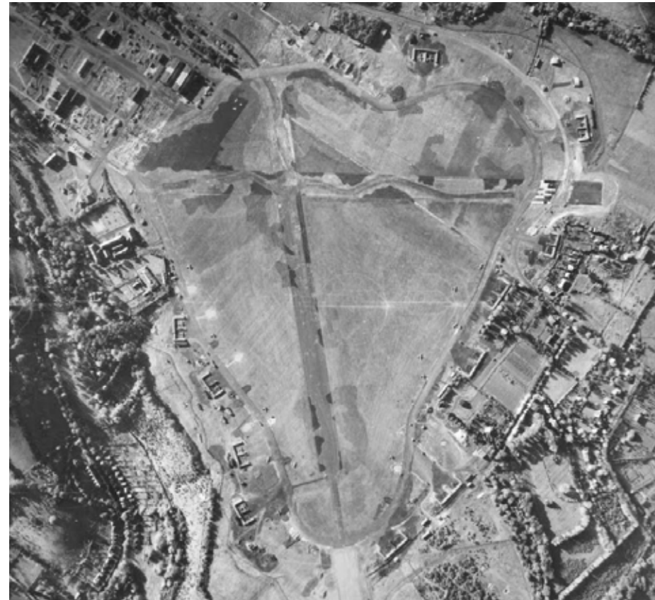
Figure 3.8 Aerial Image illustrating extent of damage during the 1940 raids on Kenley, 1941
