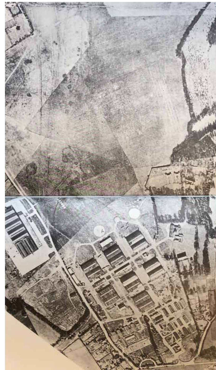
Figure 3.3 Aerial Photograph showing the completion of seven double hangars and barrack accommodation to the south. Large Bomber hangar located to the south-west of flying field, 1921.
