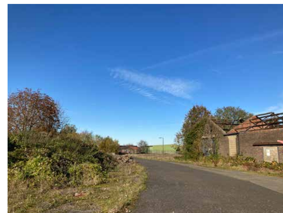
Figure 3.13 Photograph of brownfield land to the south of the airfield, including the derelict Workshops
