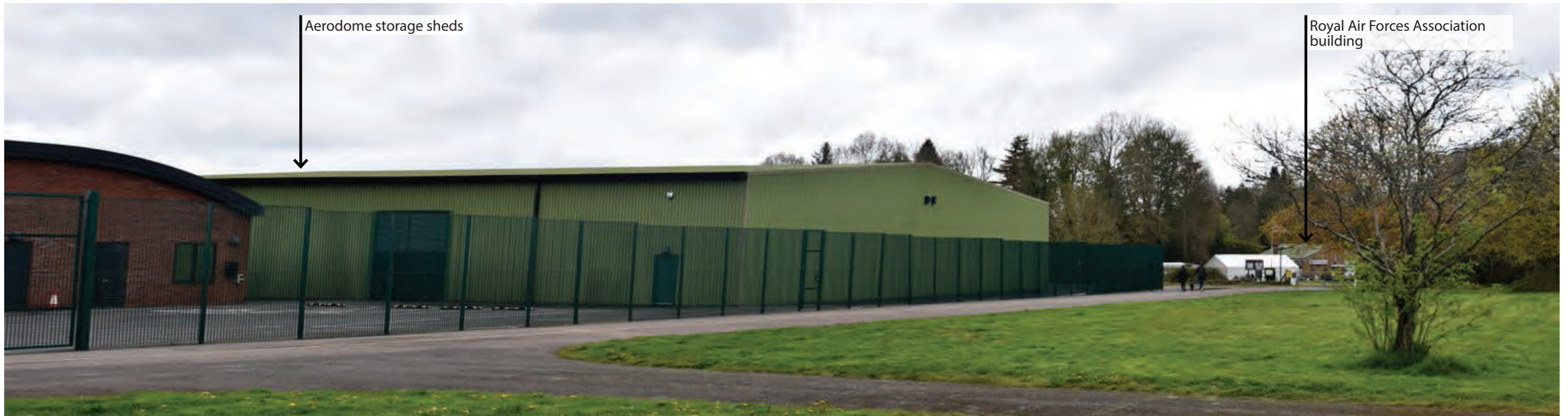
Photograph O View looking northeast towards RAF Kenley buildings
