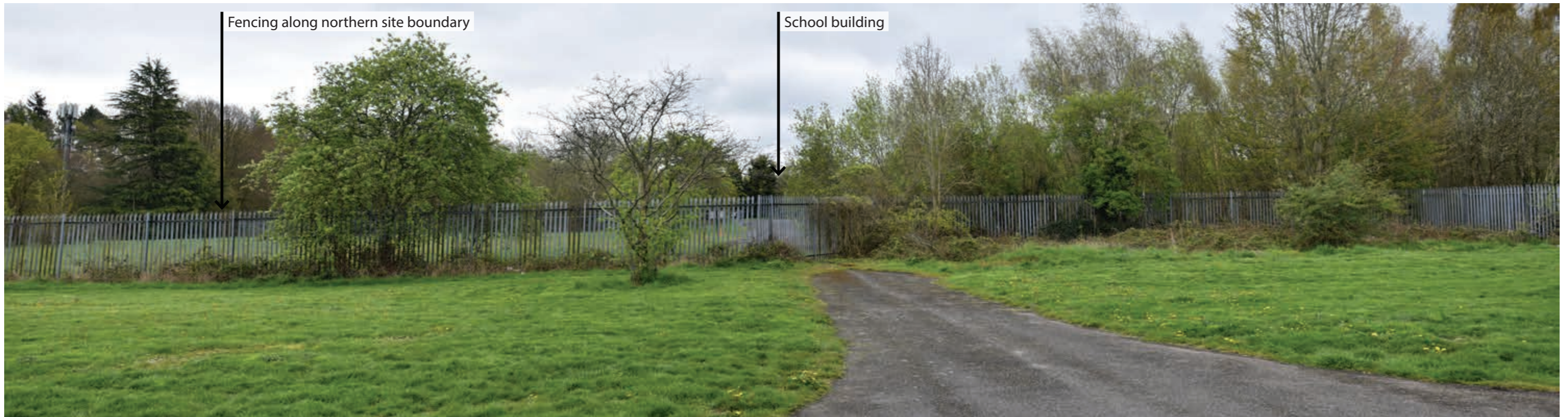
Photograph P View looking south towards school (former NAAFI building) from RAF Kenley access road
