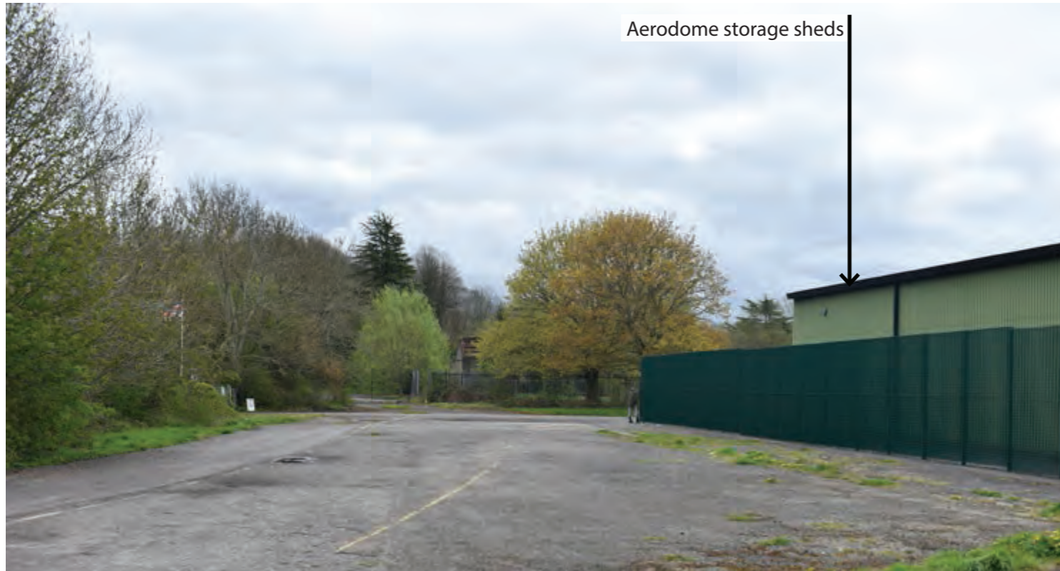
Photograph 1 View looking south towards site from airfield perimeter road (1)
