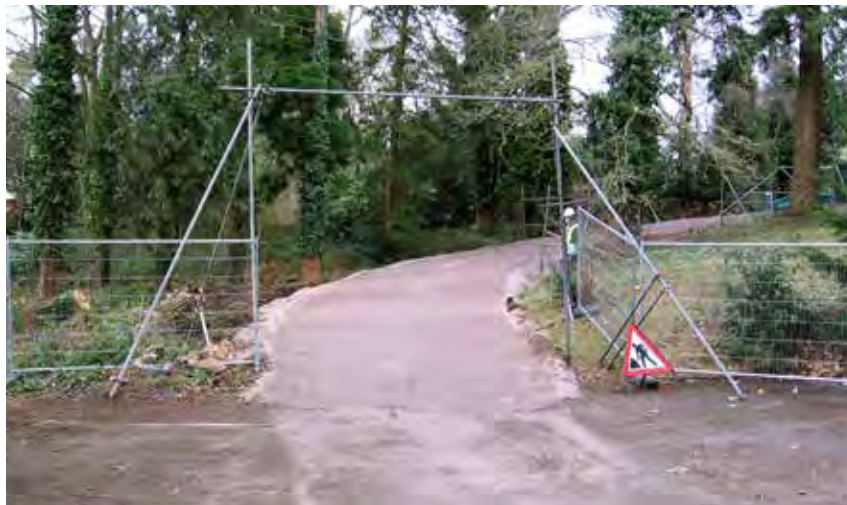
SGN 6-01 This temporary access through a woodland was height-restricted to preserve low branches that formed important screening of the new building from outside the site.
