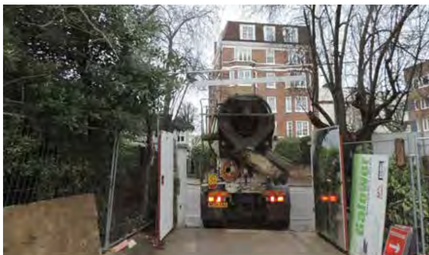
SGN 6-02 Height restriction bars are commonly used on urban sites to prevent accidental damage to low branches.
