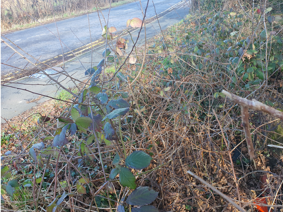
Photo 3 (View of Pipe Entering Ditch form Under Station Road)
