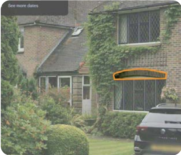
2.Arched Brick Head - Mount Avenue
