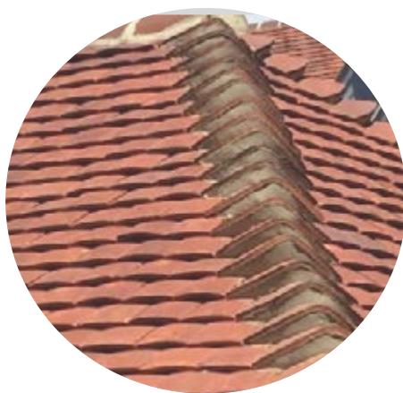
Clay Tile Roof with Bonnet Tiles
