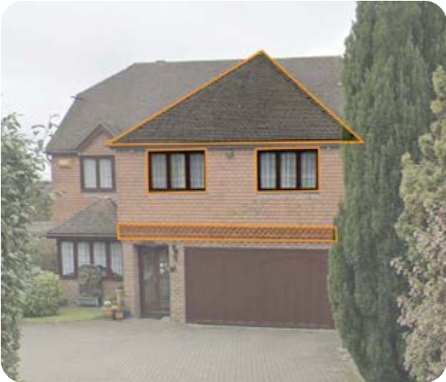
1.Tile hanging & triple pane window - Birchwood Lane
