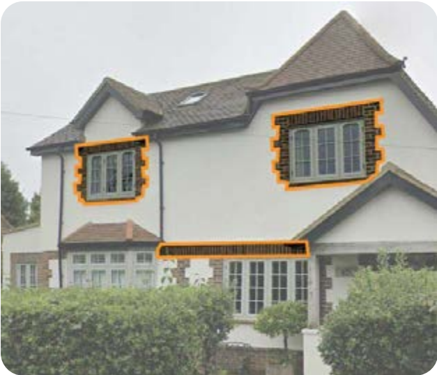
7. Brick Quoins window surround & Soldier Course - Mount Avenue
