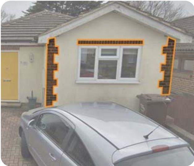
5.Brick Quoins & Brick Window Head - Sunny Rise
