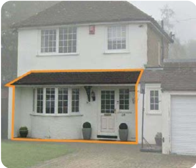
6.Mono-pitch Canopy over door & projected bay - Mount Avenue
