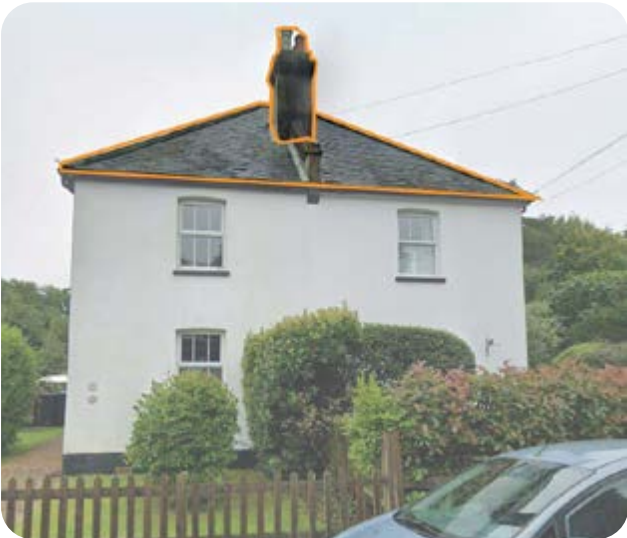
4.Slate Hipped Roof - Chimney Chaldon Common Road
