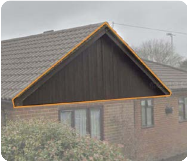
9.Feature Weatherboarding & Red multi-brick - Sunny Rise
