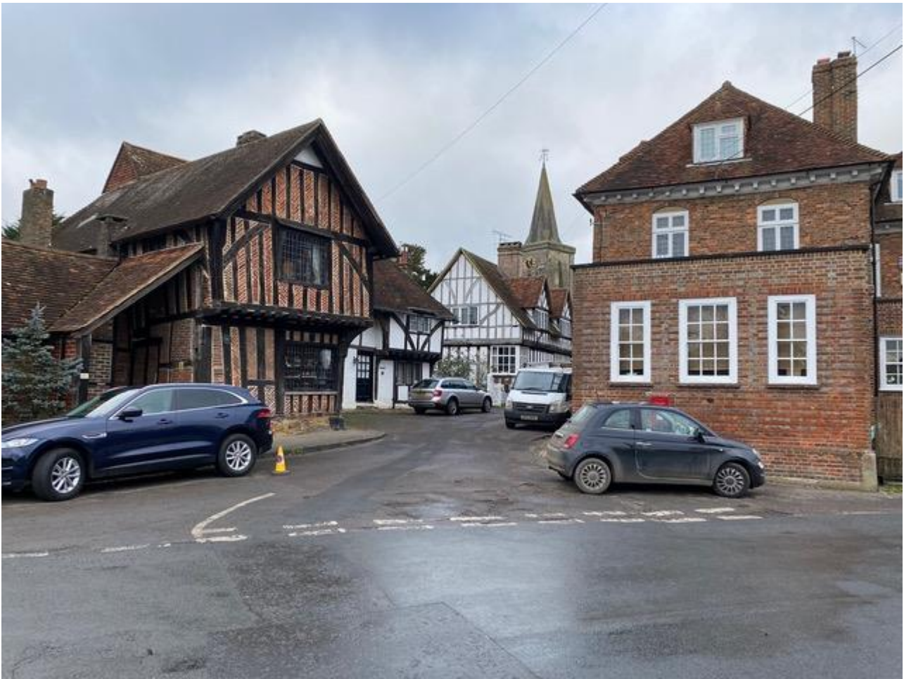
Figure 10 – General view of the core group of listed buildings in the core of the village.
