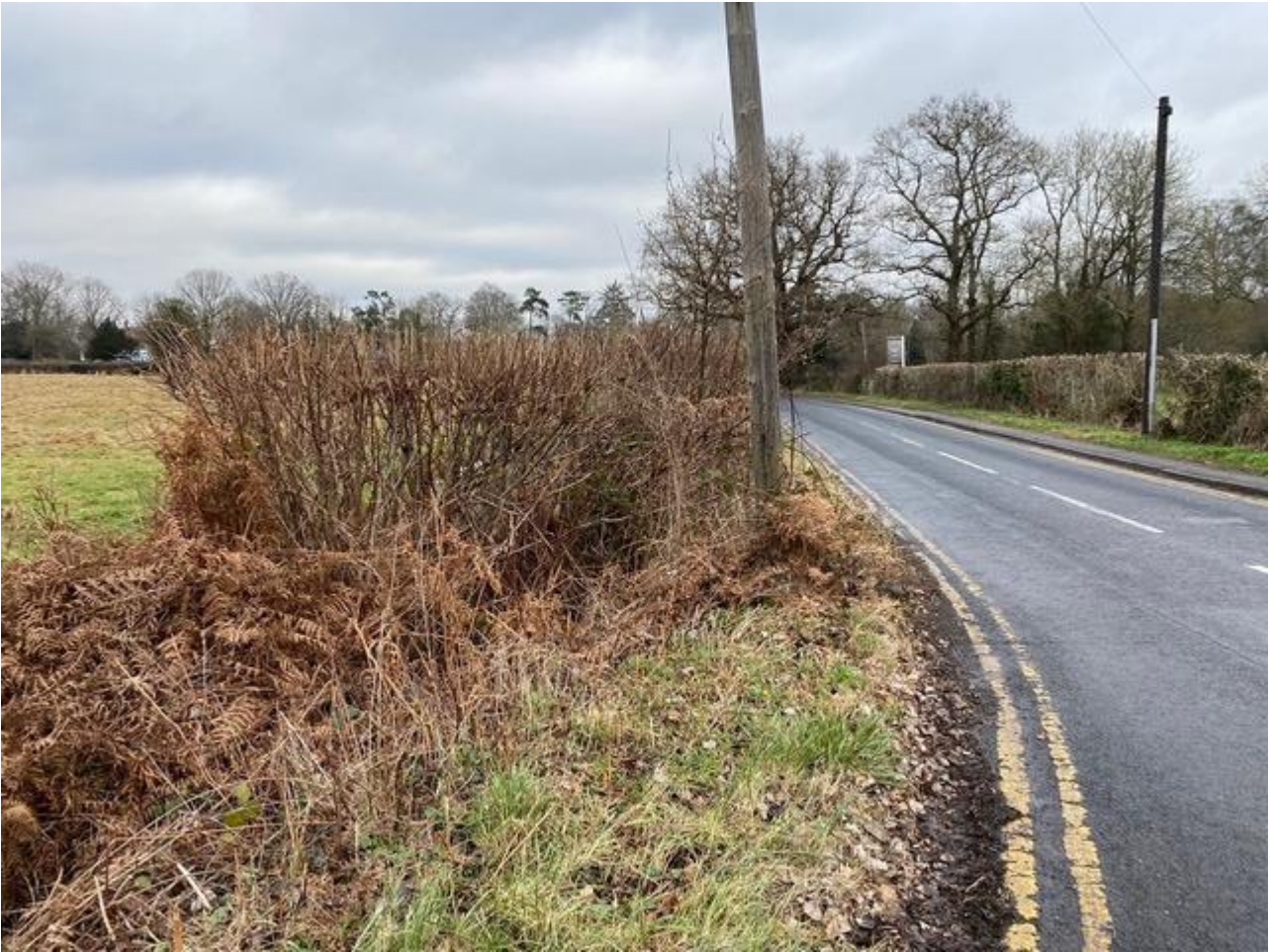
Figure 13 – Looking north in Station Road towards New Place.
