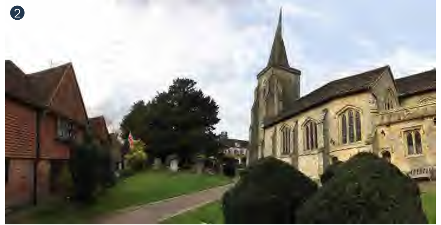
Grade II Listed Old Town House and Grade I listed Church of St Peter and St Paul
