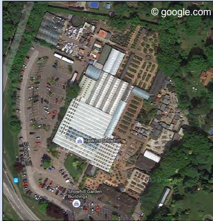
Figure A.10.12 – Snowhill Garden Centre from 2013 Aerial Photography
