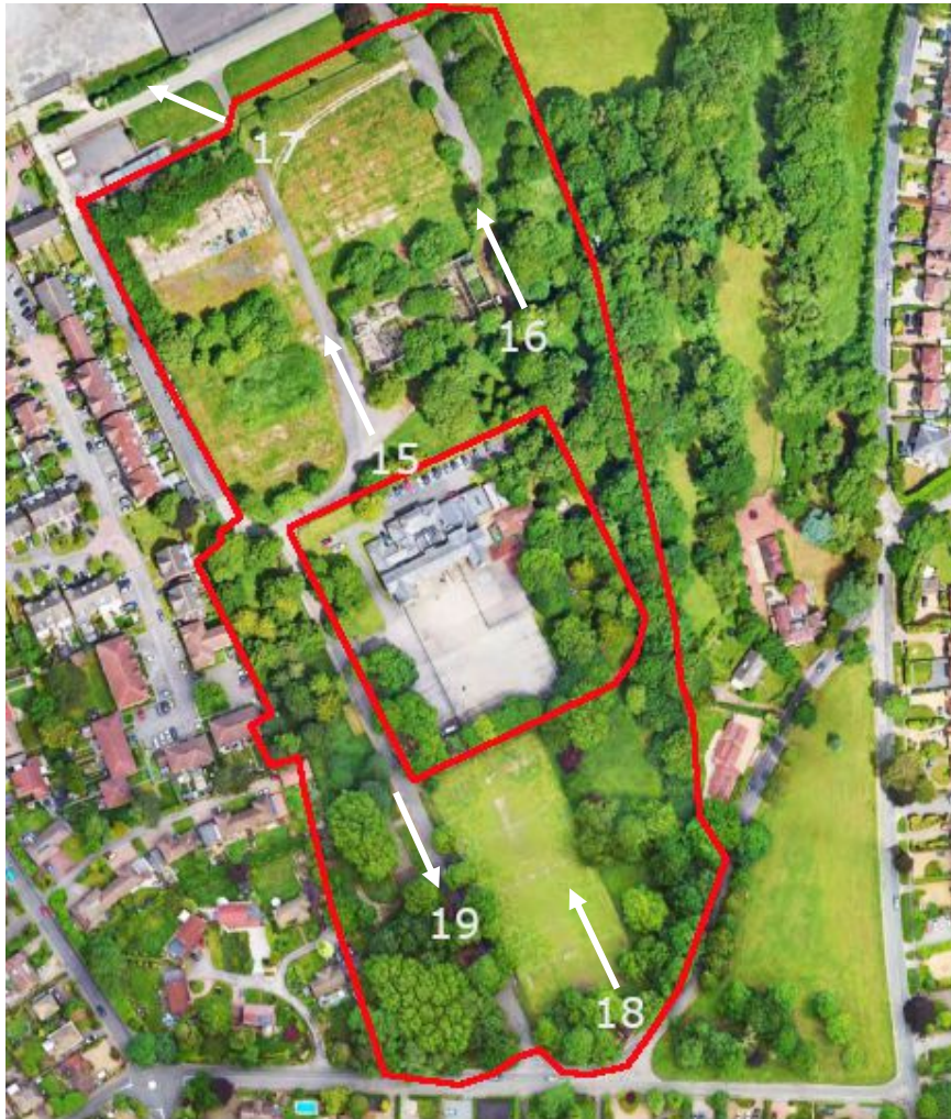
Figure 14 Aerial view of the PDA in 2022. Locations of figures 15-19 shown © Google Base Photo
