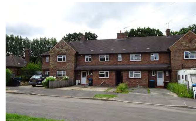
Loss of property boundaries detracts from the street appearance
