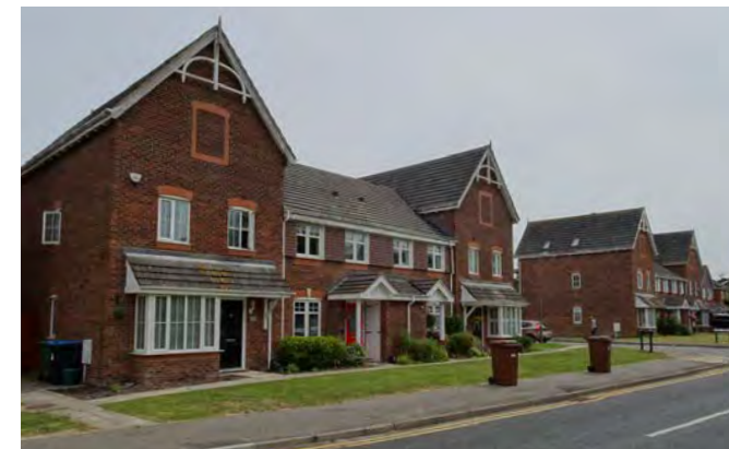
Careful positioning and form integrates three-storey development at Gray Close
