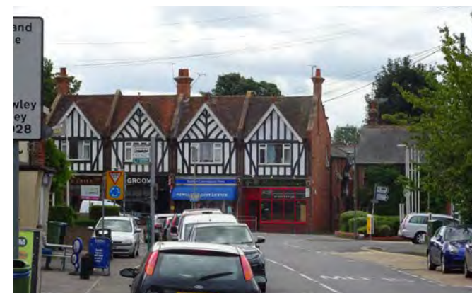
1-4 New Buildings form a focal point on the arrival into Lingfield
