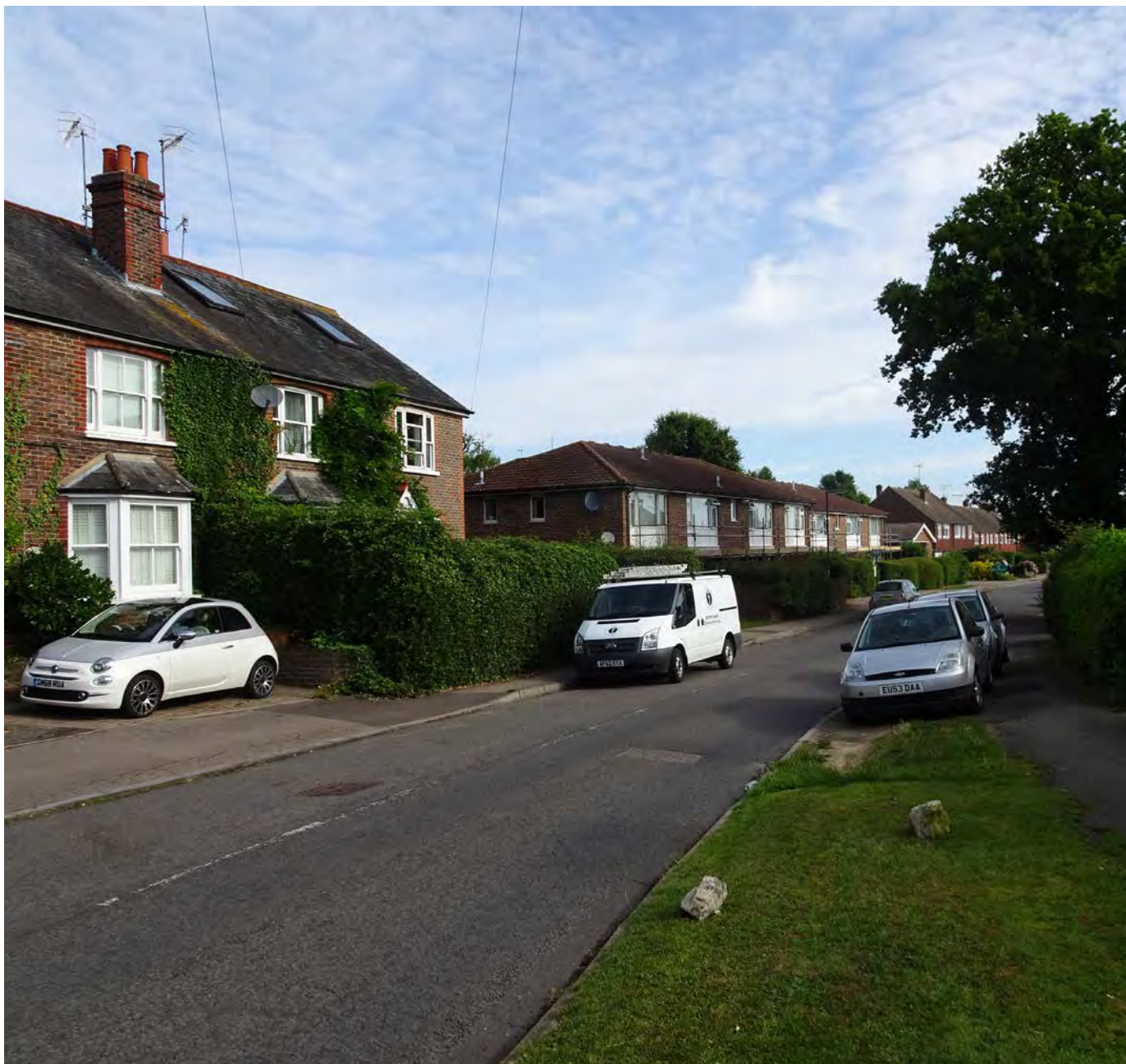
Range of building styles and architectural form.
