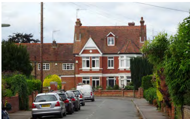
Focal point of the house at the south-west end of Mount Pleasant Rd
