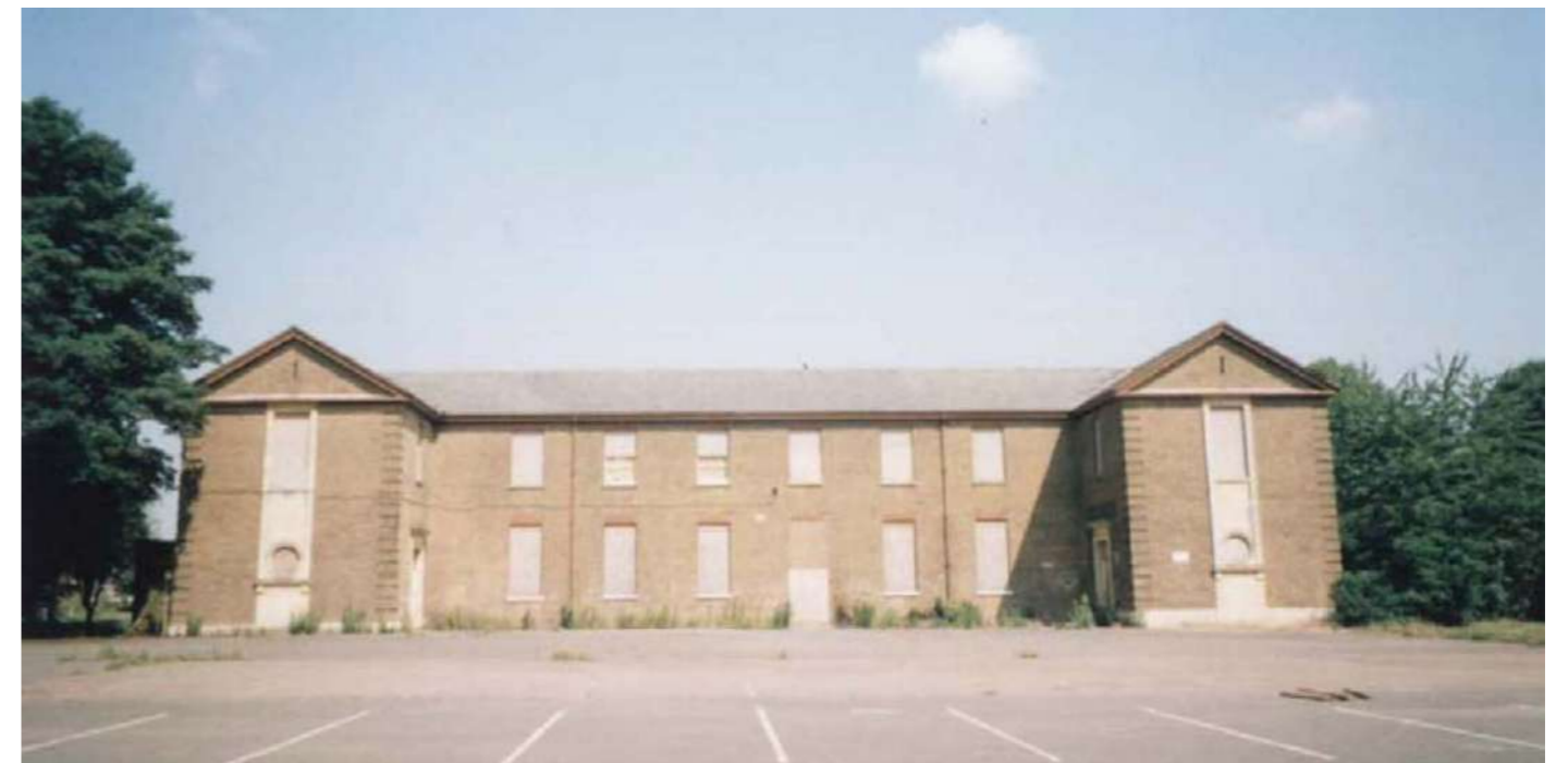
The listed Institute / NAAFI building, central to the site, presents clear character guidance of the formal military architecture.
