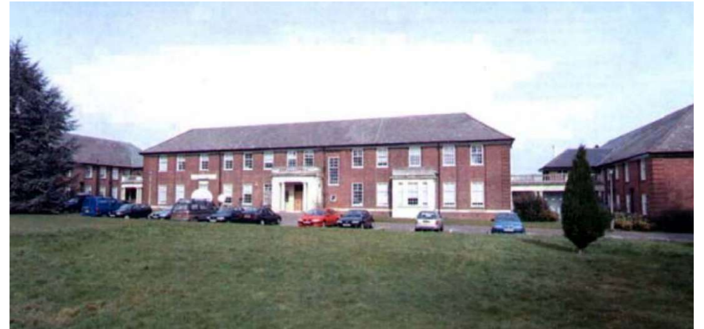
Listed Building- Officers Mess.
