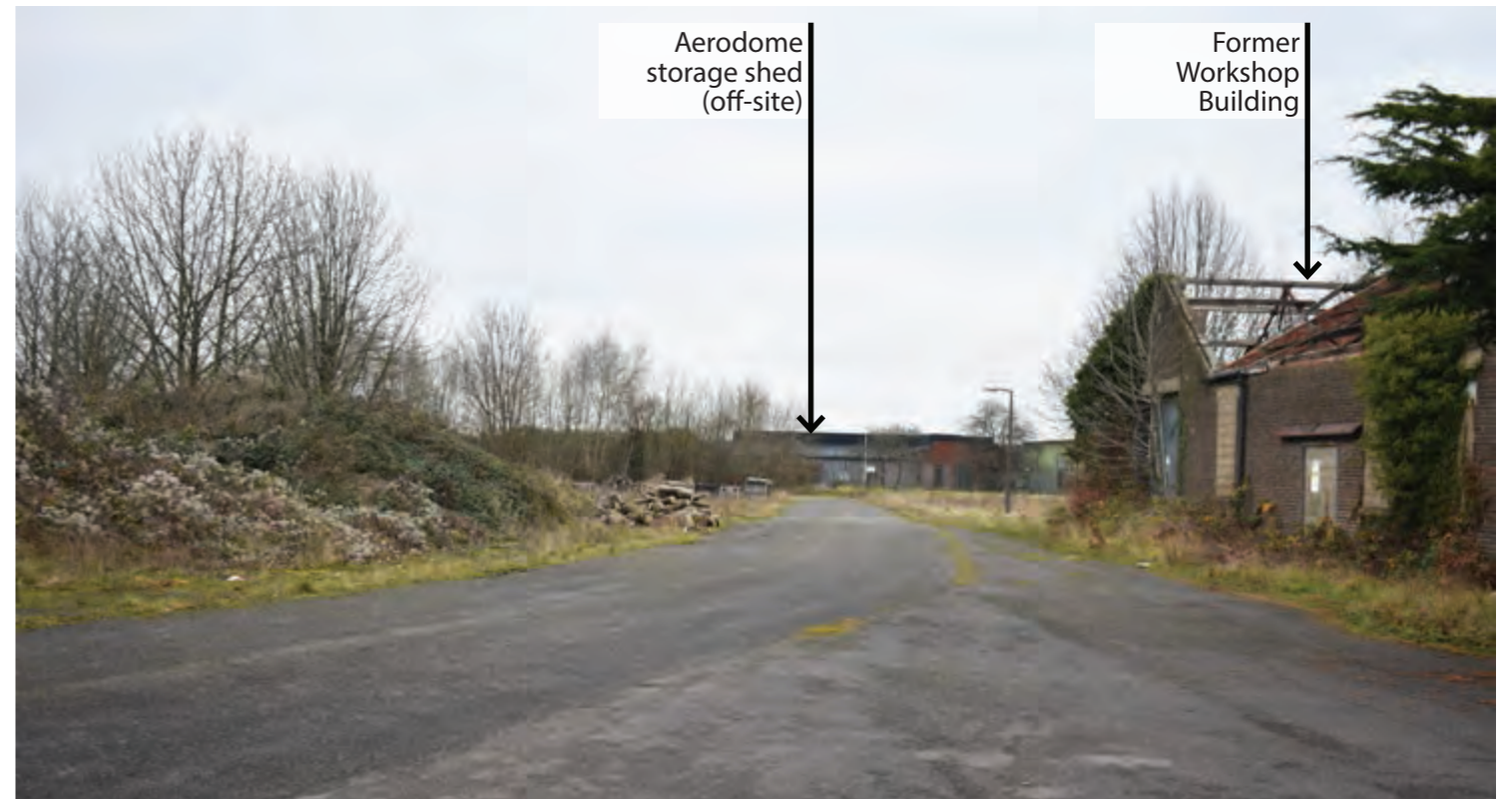
Photograph G View looking north towards airfield from track on western side of derelict workshops (Winter)
