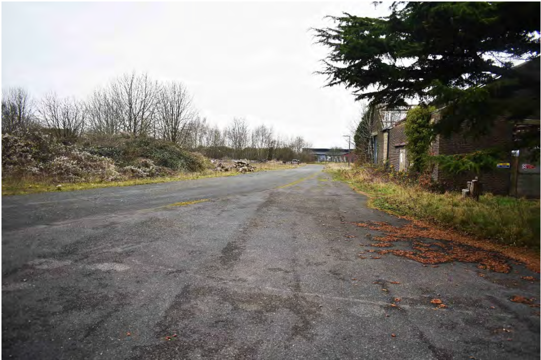
Plate 4: View of existing road, building and mounds of rubble in northern part of the Appeal Site, looking north to aerodrome (December 2021)
