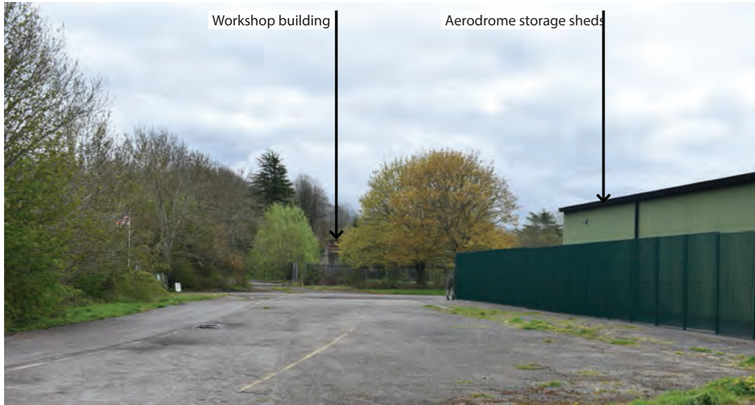
Photograph 1 View looking south towards site from airfield perimeter road (1) (Winter)
