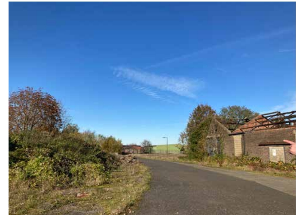
Figure 2.13 Photograph of brownfield land to the south of the airfield, including the derelict Workshops
