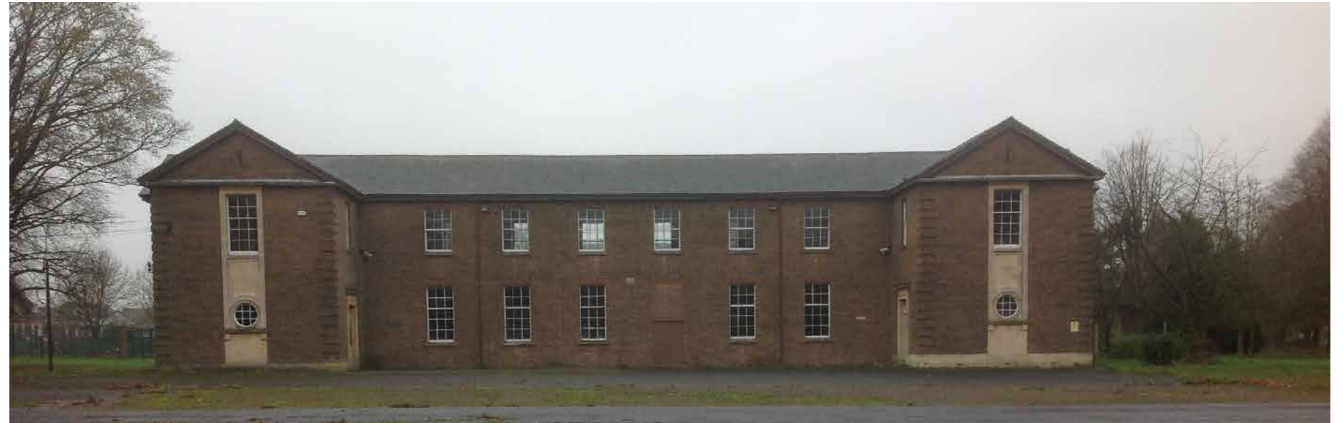
Figure 2.11 Photograph showing former Institute Building prior to recent redevelopment & conversion
