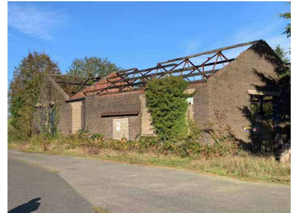
Figure 3.4 The Former Workshop, Kenley
