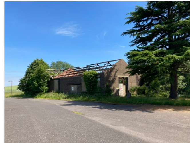
View of derelict former workshops
