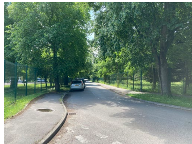
View Looking south down Victor Beamish Avenue
