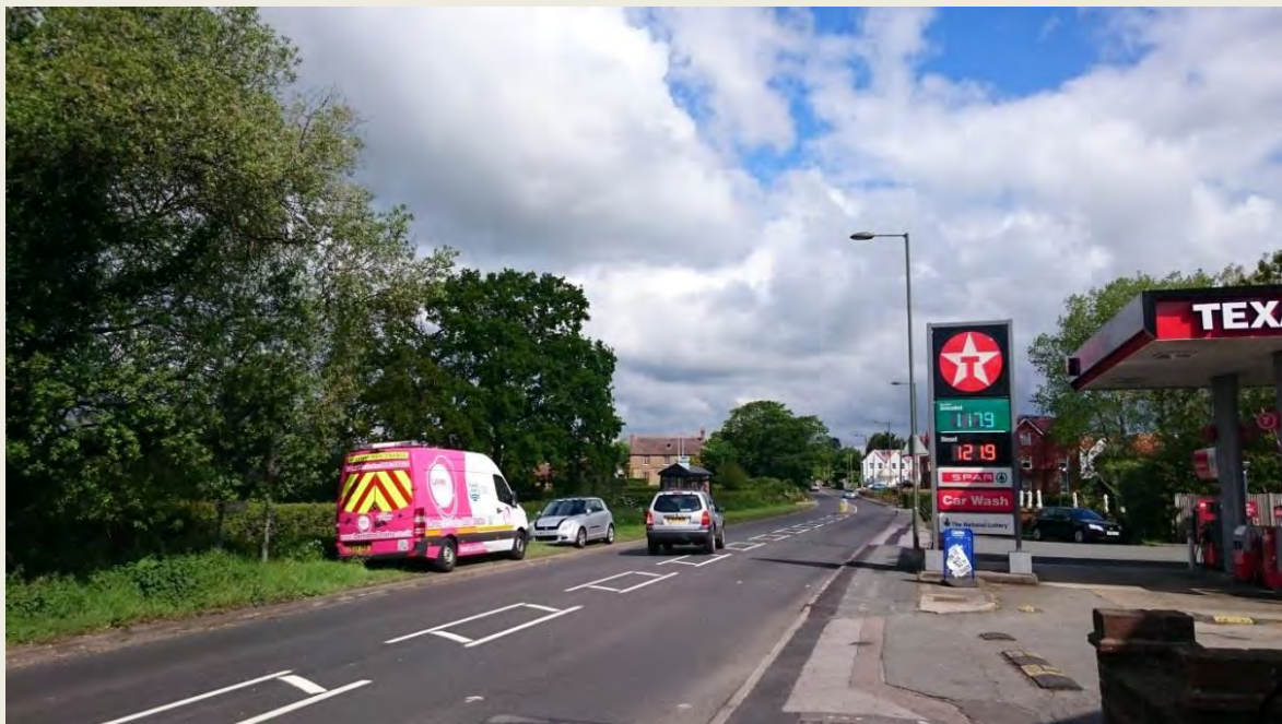
Figure D.33.3 - Development in Blindley Heath. The A22, pictured here, marks the boundary between GBA 033 and 032. The settlement is laid out on either side of the road.
