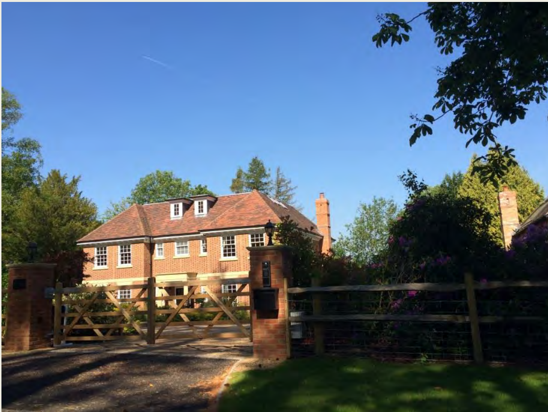
Figure D.44.3 - Large residential dwellings in the Green Belt at Dormans Park.
