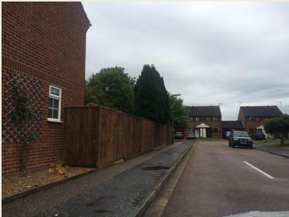
Figure D.39.3 - Residential development at Geary Close.
