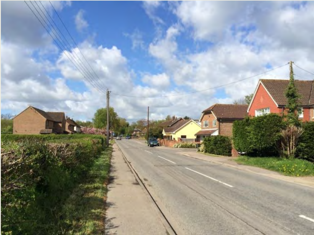
Figure D.37.5 - Residential development along Lingfield Common Road.
