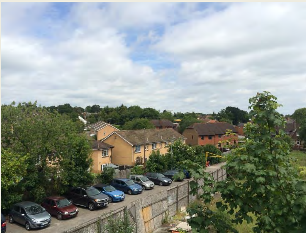
Figure D.27.4 – Some more dwellings within South Godstone, which is a settlement washed over the Green Belt.
