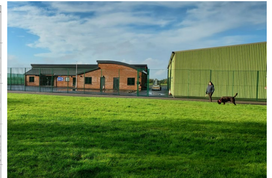
Buildings within Kenley Aerodrome with a height of 7.5m
