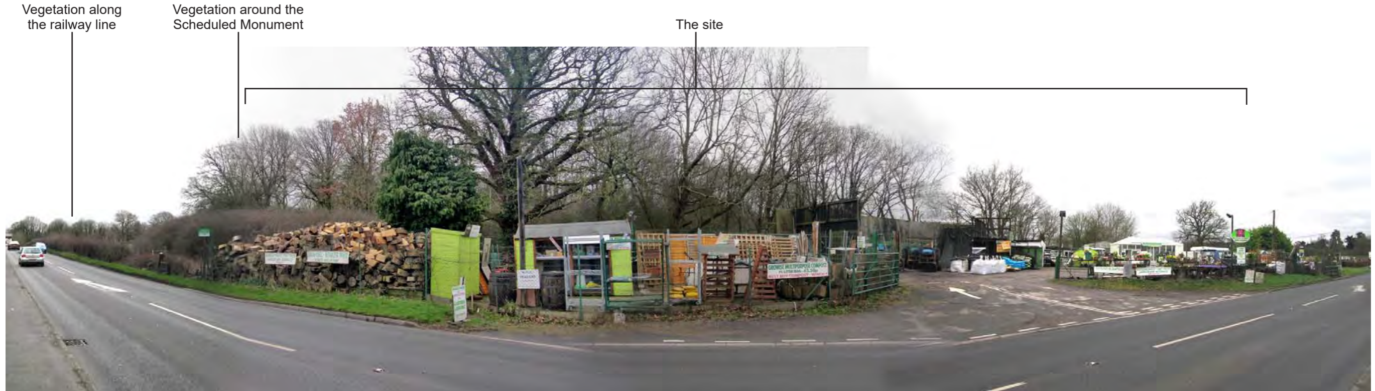
Photograph 228: View east from the A22
