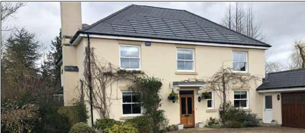
"slate" solar panels
