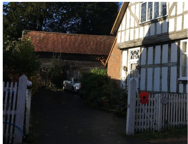
Figure 27 View of the barn from the east
